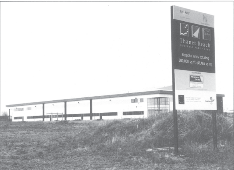
12: Industrial regeneration, as here on the Isle of Thanet, has moved from the inner city to its edge. (Edgelands)
